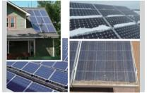
Nearby Shading, Soiling and inter-row shading
